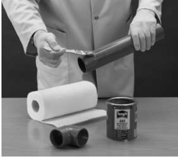
Applying the cement
