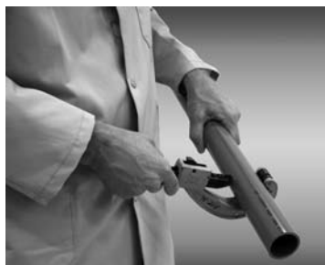
Cutting the pipe to length
