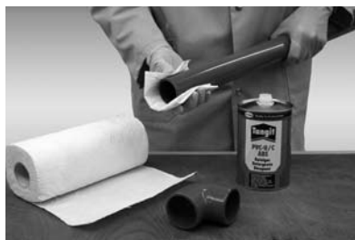
Cleaning the pipe and socket
